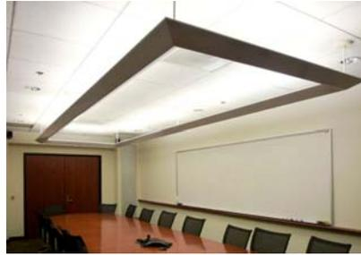
Conference room lighting system before (above) and after (right) the installation of the dc-powered infrastructure grid with LED-lighted tiles. Different color schemes and nine layers of light are available.
