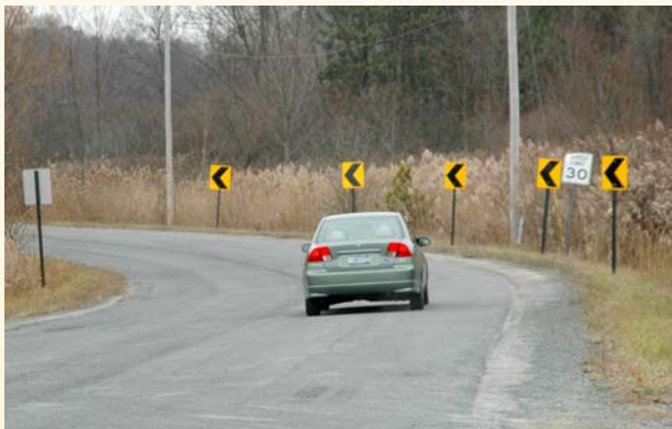
Chevron signage increases in size and spacing through the curve to give drivers the perception of a sharper curve as it is approached.
