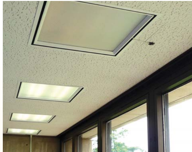
The DaySwitch turns off a luminaire when sufficient daylight is available.
