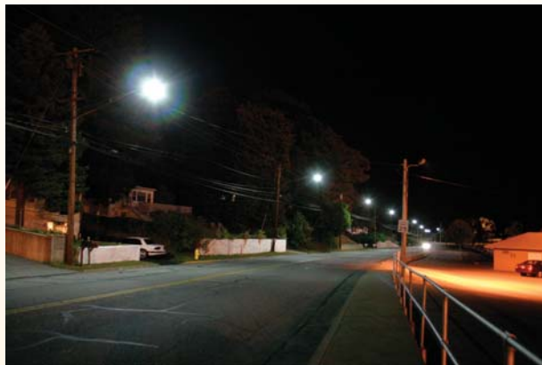
Induction lamps replaced high-pressure sodium lighting on Meridian Street in Groton, Conn. A remaining HPS lamp lights the parking area on the right in this photo.
