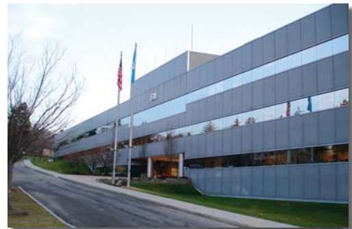
ConEd headquarters in Rye, New York (demonstration site)
