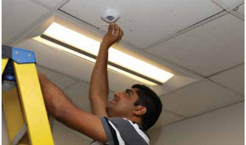
In a 25,000-sq ft commercial office on the Rensselaer Technology Park campus in Troy, NY, LRC researchers are installing LED lighting with fixture-integrated and network-connected controls. The controls are being tested in a broad-based field evaluation to compare and quantify the additional benefits that connected lighting systems offer to users. Led by LRC Director of Research Nadarajah Narendran, the LRC is investigating everything from ease of installation to user satisfaction.
