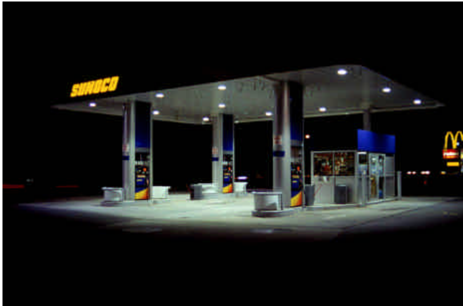
Figure 3. Photograph of the new flat-lens lighting
