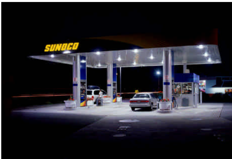
Figure 4. Photograph of the new drop-lens lighting
