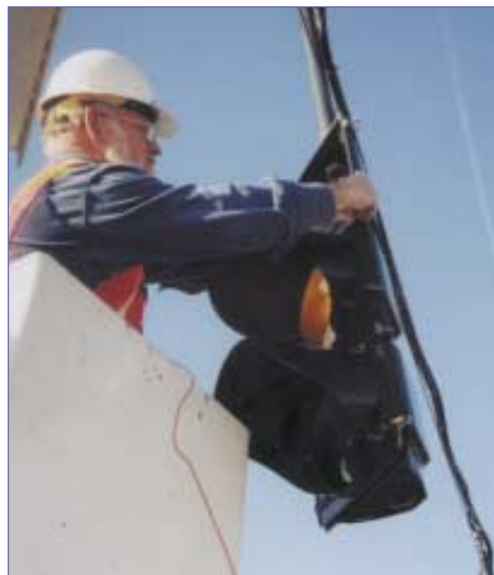
An incandescent traffic signal in Onondaga County being retrofitted with LED technology.
