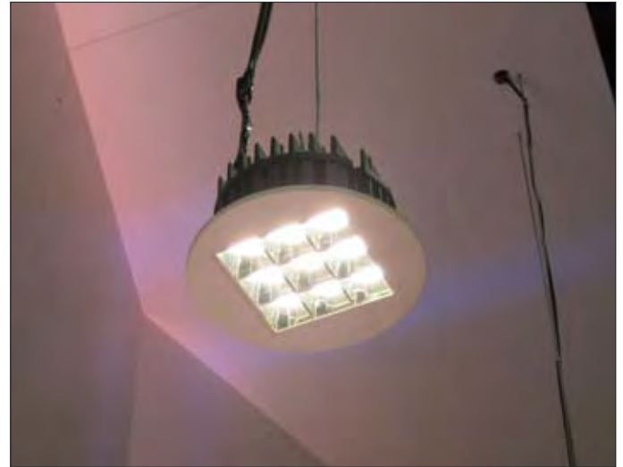
LED downlight on the Philips stand at Lightfair. Surrounding a downlight with ceiling insulation can cause considerable heat build-up inside and around the fixture, affecting the performance.
