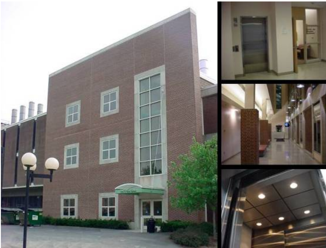
Figure 29. Exterior of the New York State Polymers Synthesis building at Rensselaer Polytechnic Institute’s main campus in Troy, NY (left), view of the elevator used for the study (top right), a view along the hallway leading to the elevator (middle right), and a view into the elevator cabin showing the existing incandescent lighting (bottom right).
