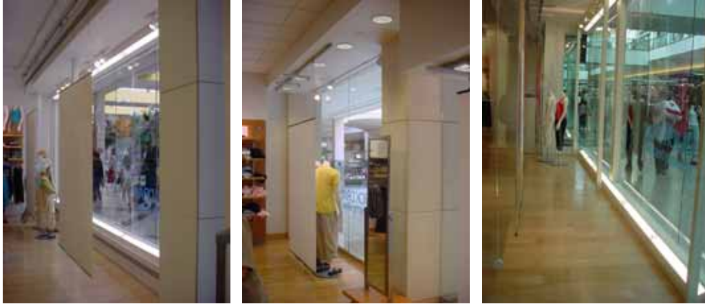
Fig. 1. Interior view of a typical window in Store 1 (left), Store 2 (center), and Store 3 (right). Note the linear fluorescent or recessed compact fluorescent luminaires for general illumination and the PAR30 halogen lamps used for accent lighting.
