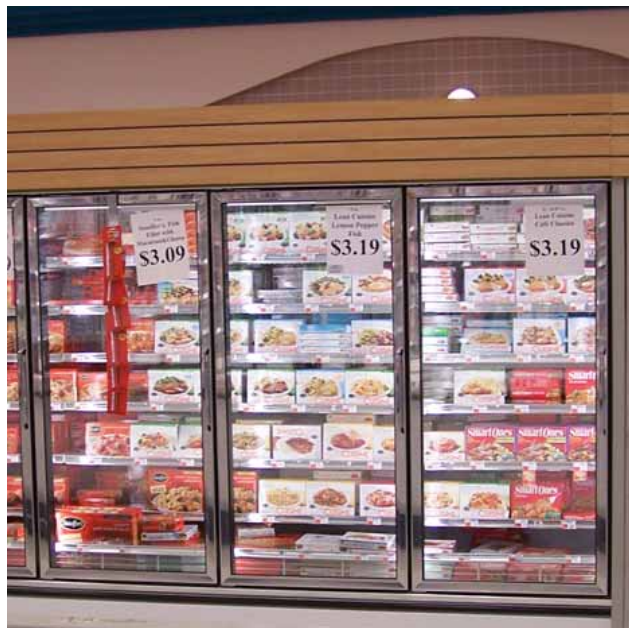
Figure 8. Existing freezers at Price Chopper.
