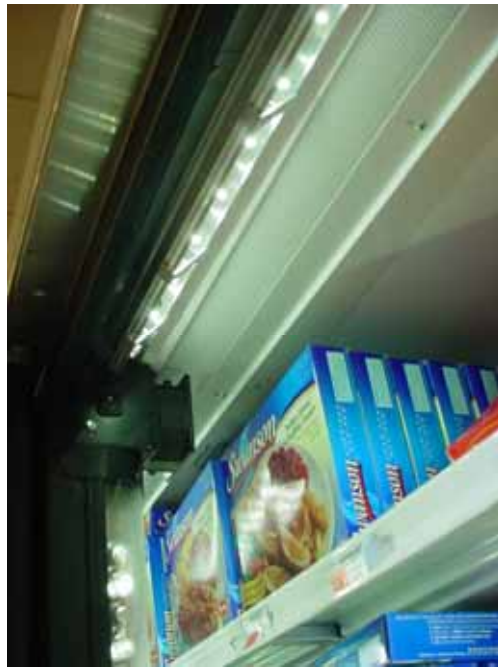
Figure 10. The top row of LEDs added to the freezer.
