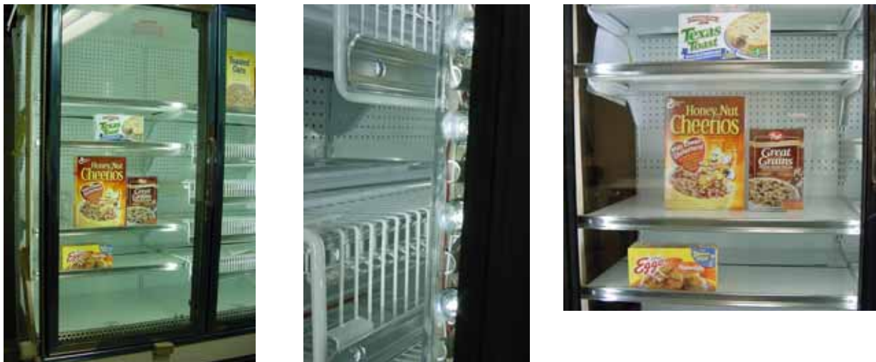
Figure 3. The LED freezer (left); close-up of the LED lighting system (center); close-up of the LED freezer interior (right).
