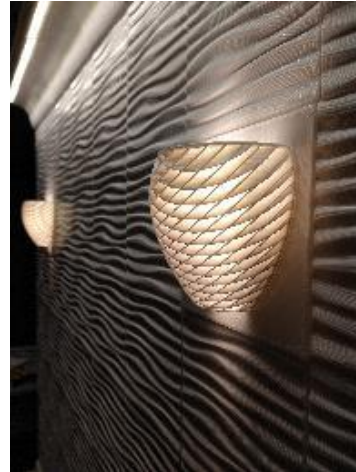
Fig. 1. (left) Prototype, scale-model sized 3D-printed interior wall with lighting (LRC photo) [11]
