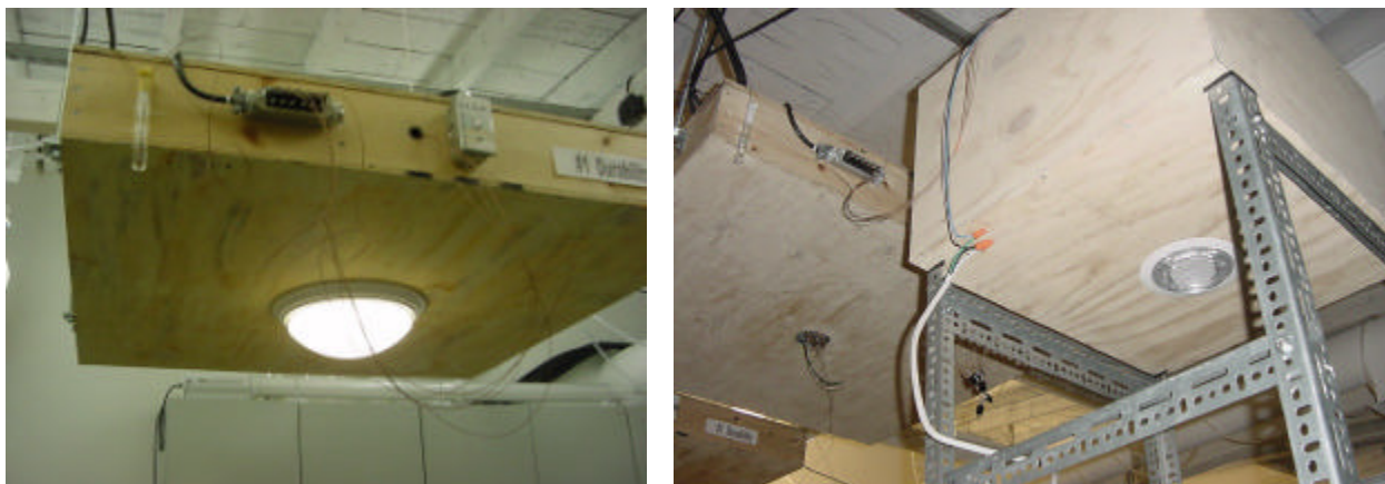
Figure 3. Temperature testing of ceiling mounted and recessed light fixtures
