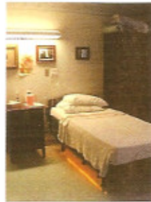
Figures 1a and 1b: Motion-sensor controlled amber LEDs installed under bed (left) and around doorway (right). The LED array under the bed provided general, low-level ambient light in the bedroom at night; illuminance levels between 10 and 15 lux were measured on the floor next to the bed. The LED array framing the bathroom door contributed approximately two to 10 lux on the floor near the door and when standing at the door frame, 10.5 lux was measured at the plane of the cornea. Notes: 1) photosensors were disconnected for the photos; 2) overhead fluorescent luminaire was kept off after installation of night-lighting. Photo: Dennis Guyon
