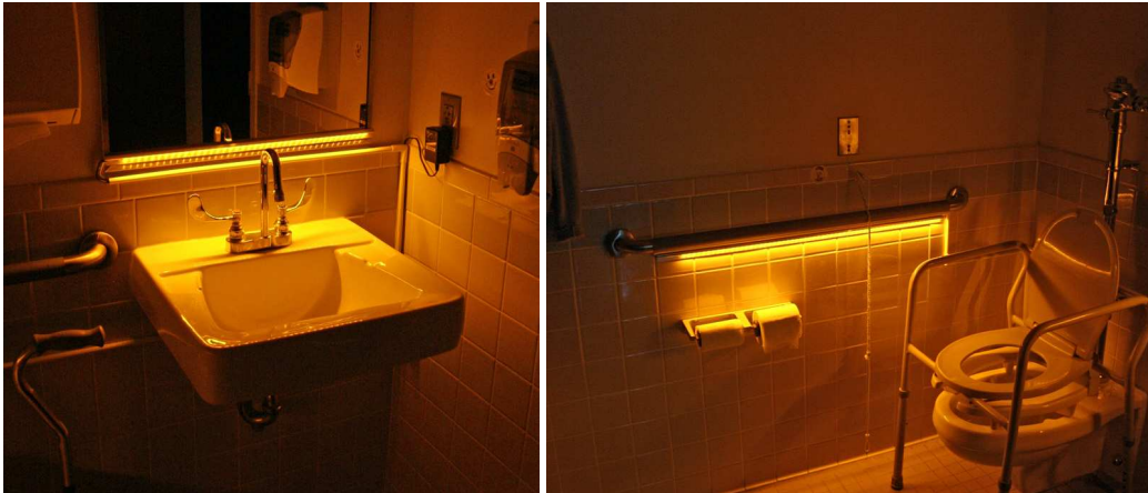
Figures 3a and 3b: Amber LEDs installed at sink (left) and toilet (right) areas.
