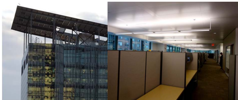
Figure 2. The Edith Green-Wendell Wyatt Federal Building exterior, west facade showing sunlight-attenuating reeds, (left) and interior (right).
