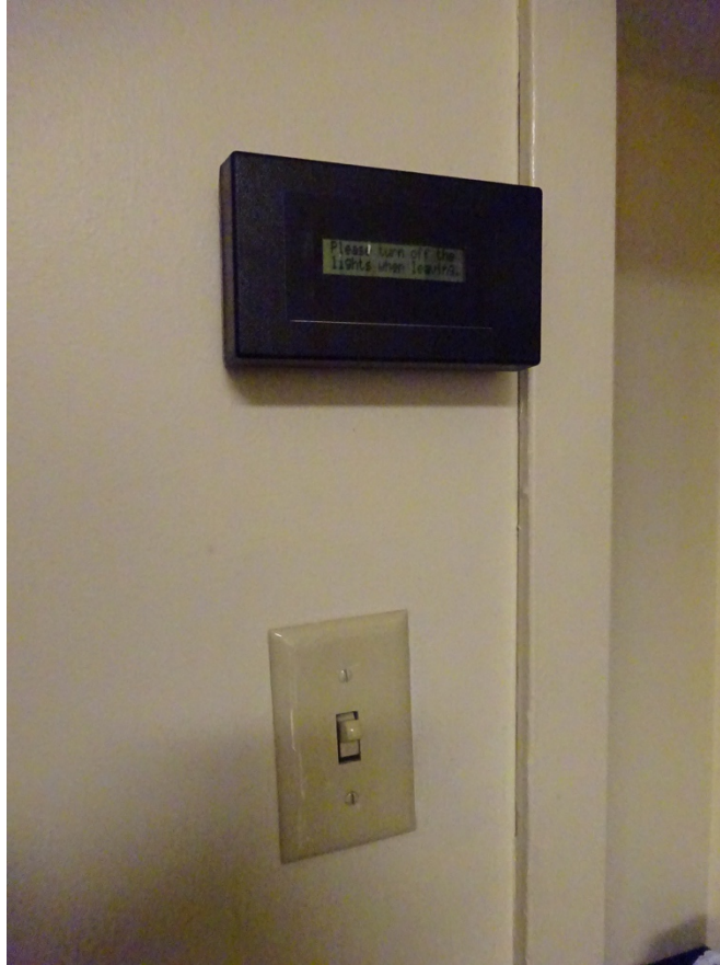
Figure 5: Static message unit mounted to wall.
