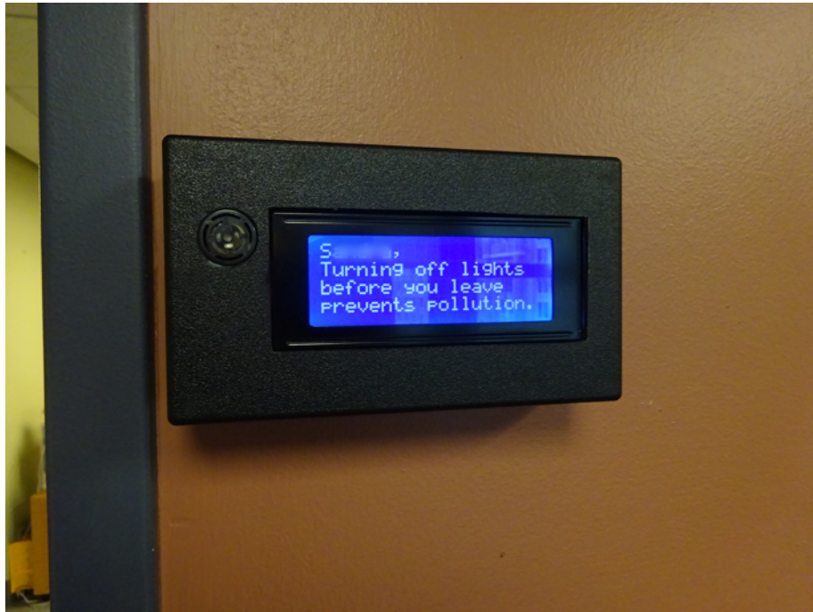
Figure 3: A dynamic message device mounted above a light switch. The occupant's first name is blurred in the photo for anonymity. The circle to the left of the display is the range finder. The black case is 5.75 inches by 3.25 inches.
