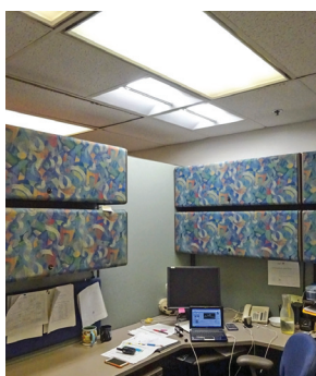
Lighting intervention. (top) An office worker uses a desktop luminaire; (bottom) CREE PoE SmartCast 2x2 troffers installed in an office workspace.
