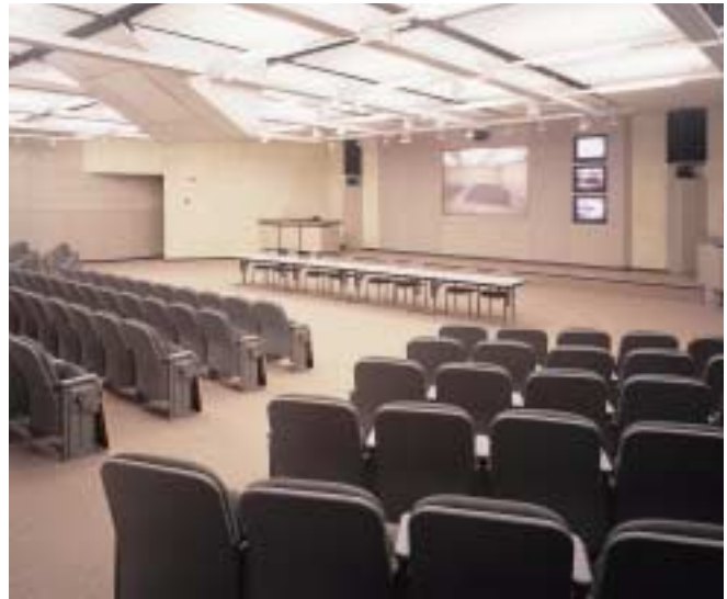
Indirect lighting, luminaires nearest to screen turned off (looking toward front)
