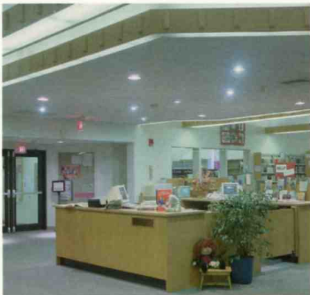
Circulation desk before retrofit. (Note the obvious high-angle glare from the CFL reflector lamps.)
