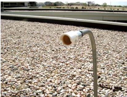
*The roof-mounted photosensor faces north.*
