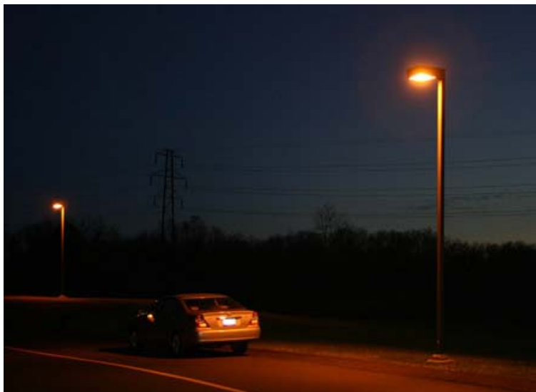
Figure 7. Most outdoor lighting systems use high pressure sodium lamps
