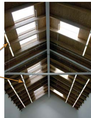
Conventional translucent skylight on south slope of the roof
