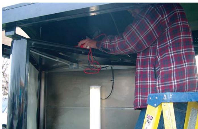
The fluorescent luminaire is mounted vertically on the back wall of the light box (shown during retrofit kit installation).
