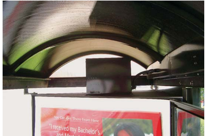
The enclosure for the batteries and controller is mounted above the light box (arch-shaped concealing plate removed for photo).
