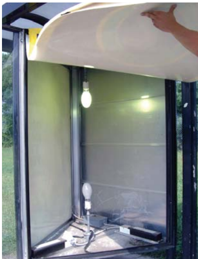
Before retrofit, mercury vapor lamps backlight the advertising posters.
