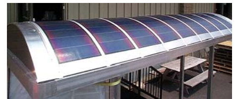
PV panels conform to the shape of the roof.
