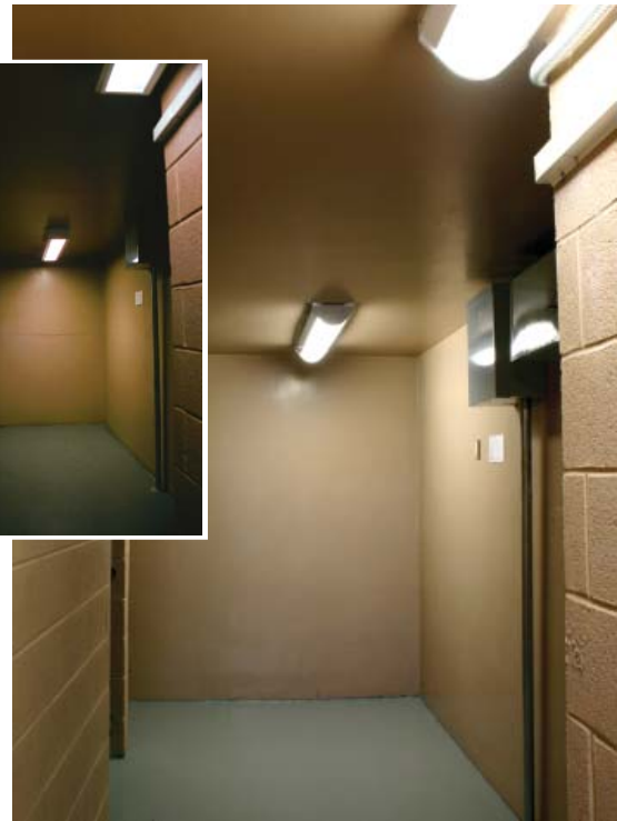
Before (inset) and after Occu-smart retrofit, Rivercross staircase, New York
