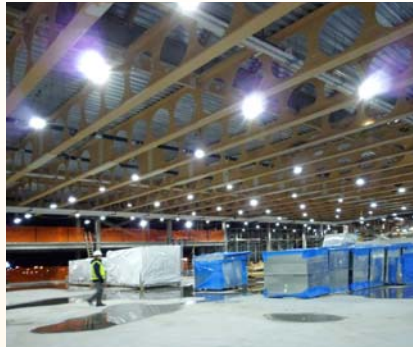
Temporary LED construction lighting was installed in the 50,000 ft 2 (4625 m 2 ) gymnasium at the new campus of New York City's Police Academy. Ceiling height was 27.5 ft (8.4 m).
