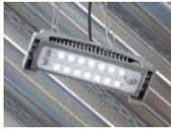
Temporary LED construction lighting was installed in the 50,000 ft 2 (4625 m 2 ) gymnasium at the new campus of New York City's Police Academy. Ceiling height was 27.5 ft (8.4 m).
