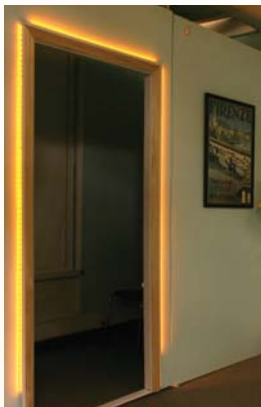
LEDs give horizontal and vertical cues around the doorway.
