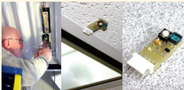
The DaySwitch installs in two easy steps. First, the microcontroller is installed inside the luminaire to switch the lamps on and off. Second, the photosensor is connected to the microcontroller via wires and is mounted outside the luminaire to measure daylight levels in the space.
