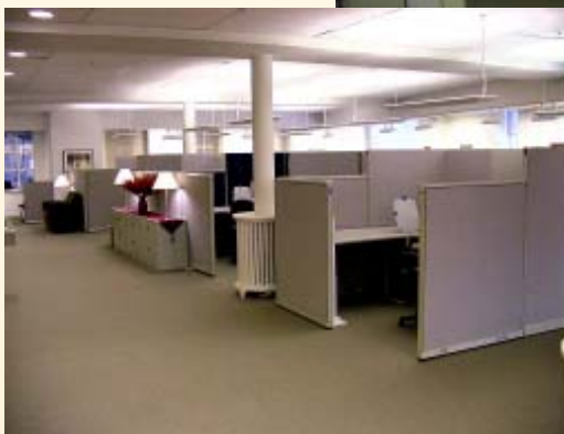
Dimming Control: Direct/indirect luminaires suspended over the center of each cubicle, together with wall-washing. The direct component could be dimmed by the occupant of the cubicle.
