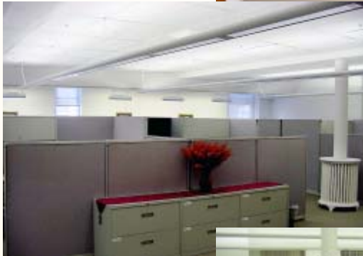
Best Practice: A linear system of direct/indirect luminaires together with some wall-washing fixtures
