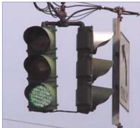
Detail of a green LED signal.
