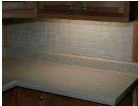
24 in. high-power LED “warm white” fixture Average illuminance: 119 lux Minimum illuminance: 37 lux Meets recommendation for critical tasks? No Uniformity on counter: 3:1
