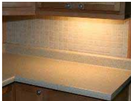
18 in. xenon linear fixture Average illuminance: 204 lux Minimum illuminance: 72 lux Meets recommendation for critical tasks? No Uniformity on counter: 3:1
