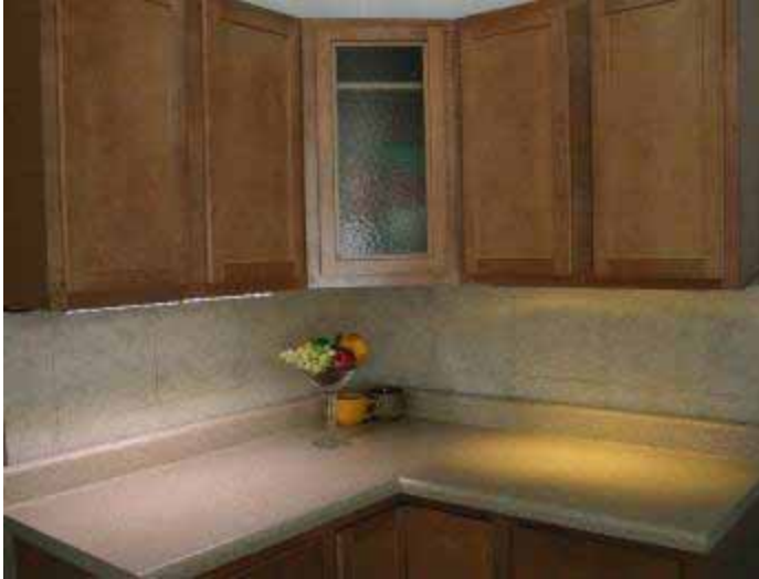
Each cabinet features an LED fixture. The fixture on the right provides poor uniformity and distribution, creating a central pool of light on the counter, poor lighting on the backsplash, and dark areas on the counter.
