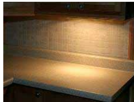
12 in. halogen two puck light bar Average illuminance: 322 lux Minimum illuminance: 90 lux Meets recommendation for critical tasks?: Yes Uniformity on counter: 4:1
