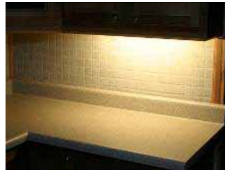
16 watt T4 linear fixture Average illuminance: 408 lux Minimum illuminance: 140 lux Meets recommendation for critical tasks?: Yes Uniformity on counter: 3:1
