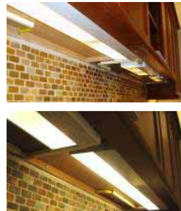
Above: Forward mounting of fixtures, facing backsplash.
