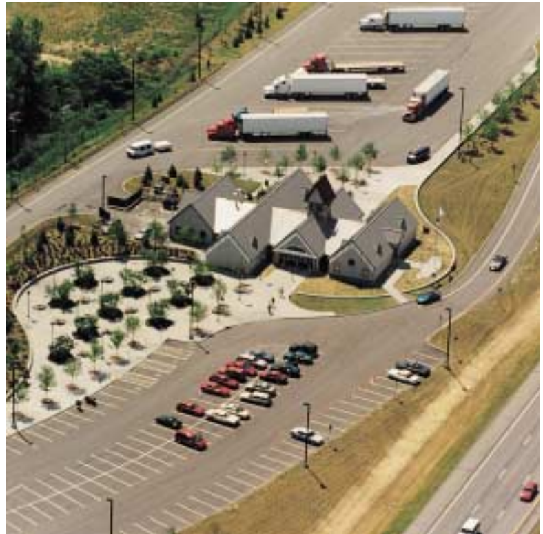
Clifton Park Rest Area, looking south
